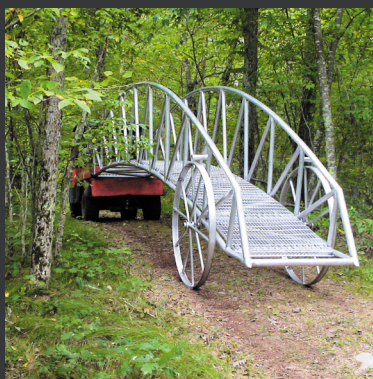
Wheelbridge, aluminum, on the Eightmile River, removable in the event of flooding, 2009 (8 meters)
