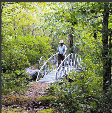
Wheelbridge, aluminum, on the Eightmile River, removable in the event of flooding, 2009 (8 meters)
