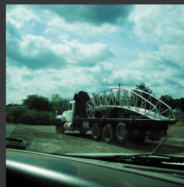
Wheelbridge, aluminum, on the Eightmile River, removable in the event of flooding, 2009 (8 meters)
